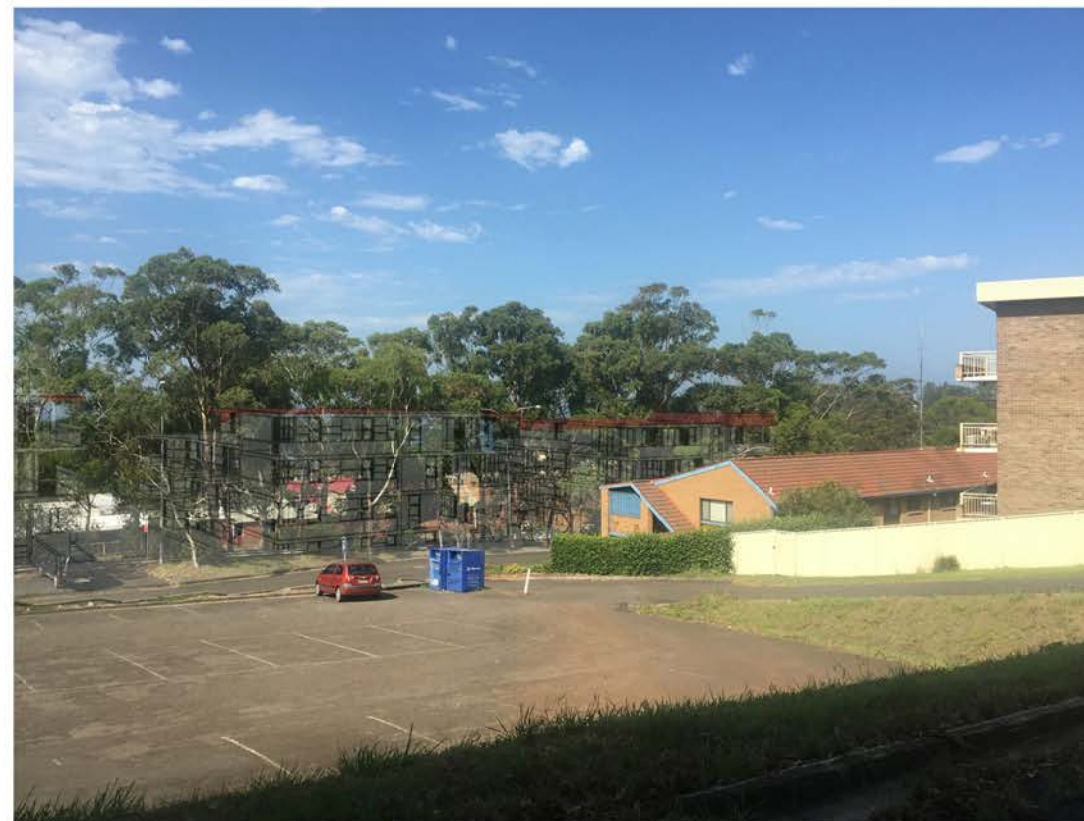
VIEW 01 - FROM TOP TIER OF PARKING LOT ACROSS FROM SUBJECT SITE FACING EAST
